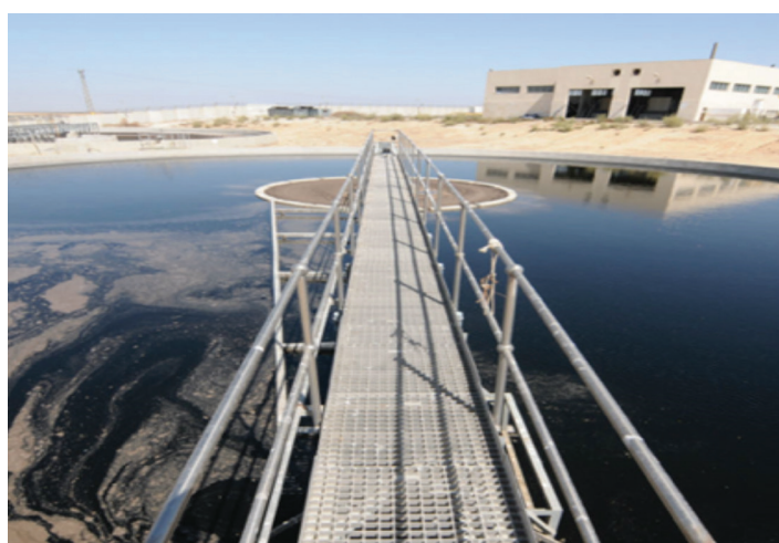
The Wastewater Treatment Plant, Bnei Shimon Regional Council (source: Mey Sheva Regional Corp. for Water and Sewage Ltd.)
