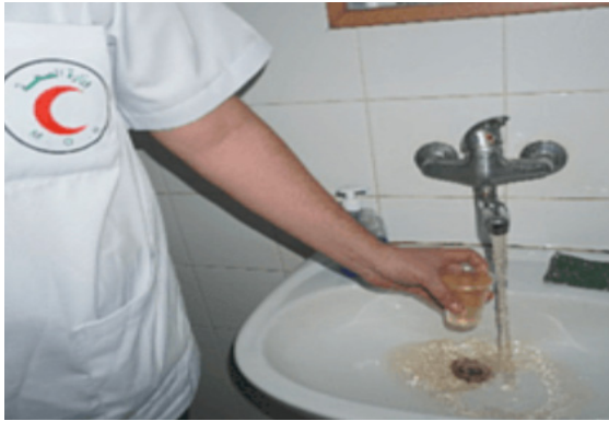
Figure 5: A member of the medical staff shows rusty water coming through the water system, Shifa Hospital, Gaza, November 2018 (Source: OCHA) (25)
